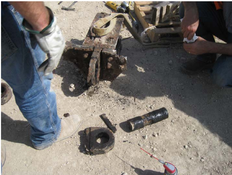
Figure 5-4 Castings, Hinge Plates, and Pin
