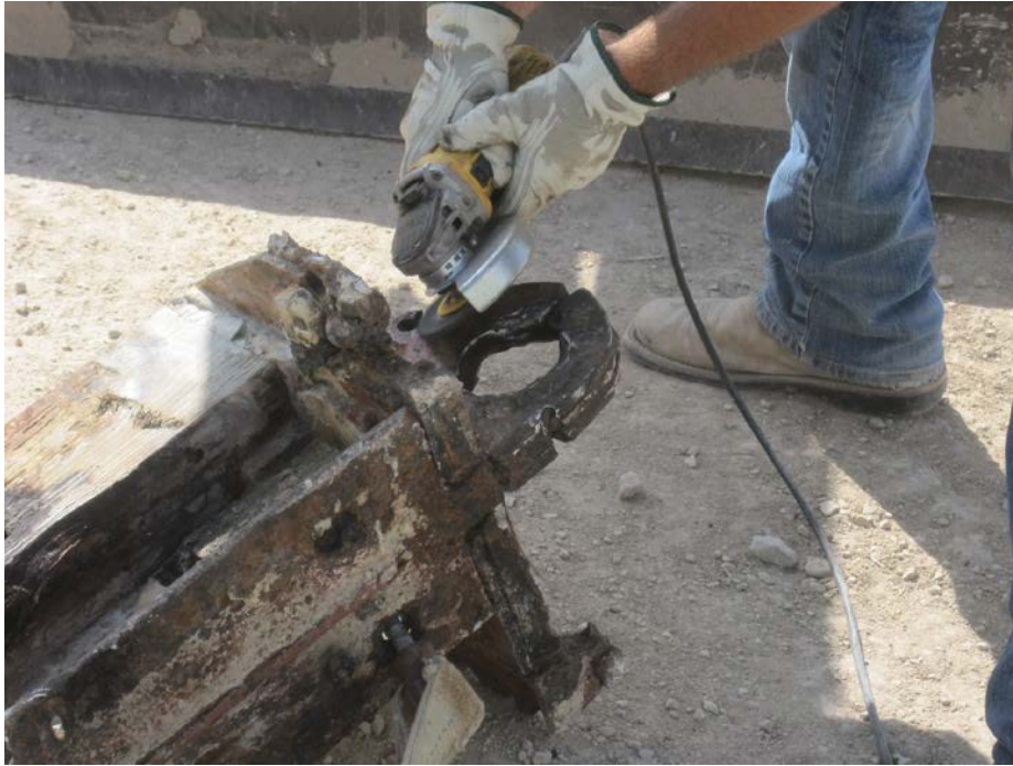
Figure 5-5 Wire Brushing to Clean Hinge Plates
